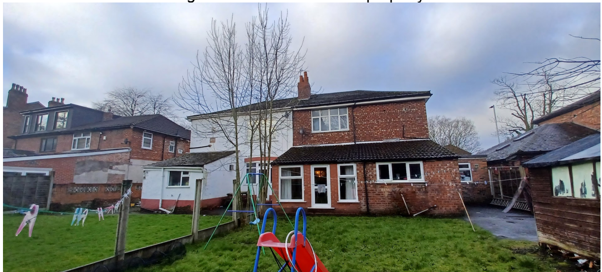
Figure 5. Shared boundary with No.185 Withington Road.
