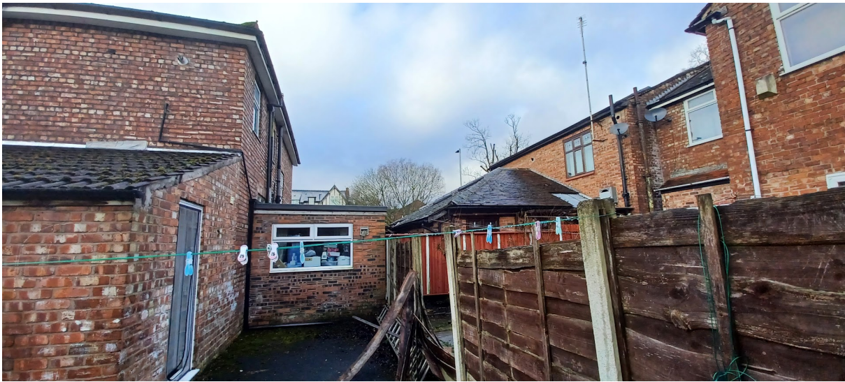
Figure 6. Shared boundary with No.181 Withington Road.
