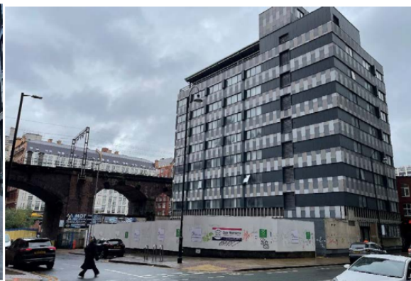
View north-east along Charles Street and towards Lass O' Gowrie Public House from junction with York Street
